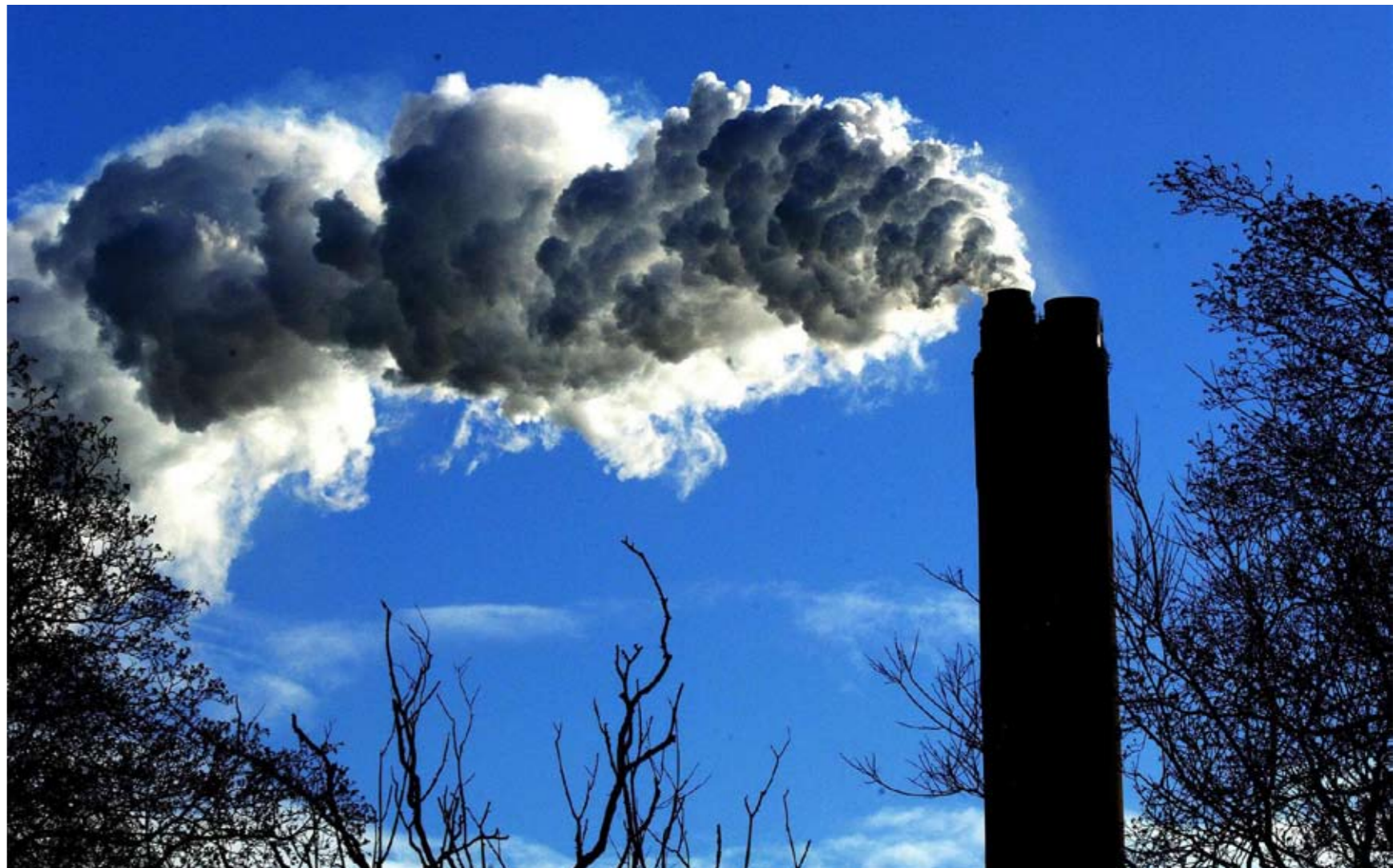
Sachs: 'It is hard to see how greenhouse gas emissions can be stabilised by mid-century without a decisive adoption of CCS technologies in coal-fired plants around the world'
